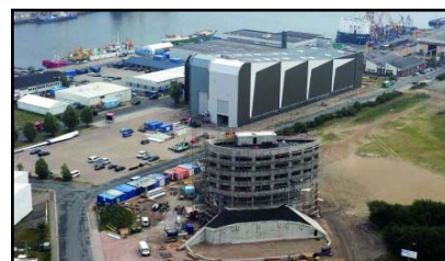
Test Center for 90m Blades Fraunhofer IWES Bremerhaven
