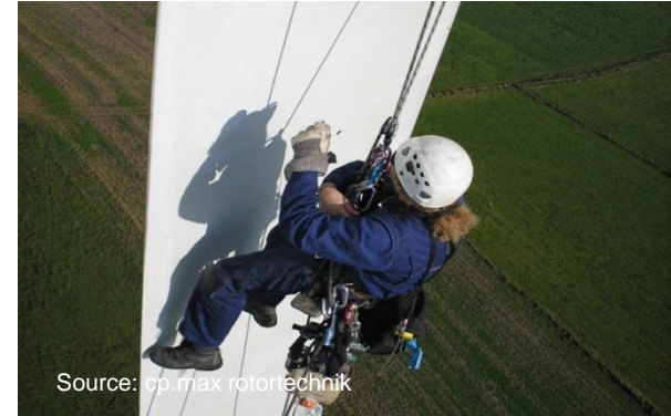
Inspection of rotor blade
