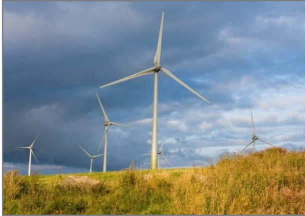
Wind farm Kryštofovy Hamry, Czech Republic
