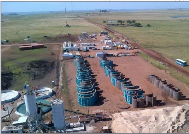
Wind farm Peralta, Uruguay, concrete factory+ prefabricated tower segments
