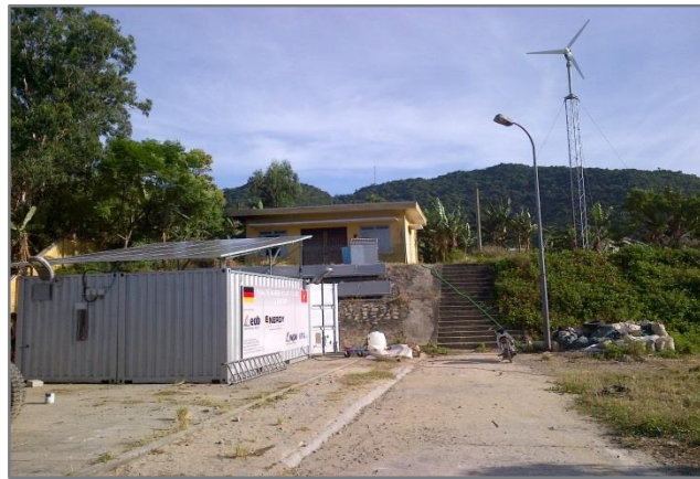
Pilot station in Vietnam for drinking water abstraction & generation of electric power
